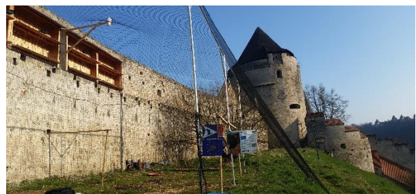
Fig. 2: New breeding facility at Burghausen; Photo J Fritz
